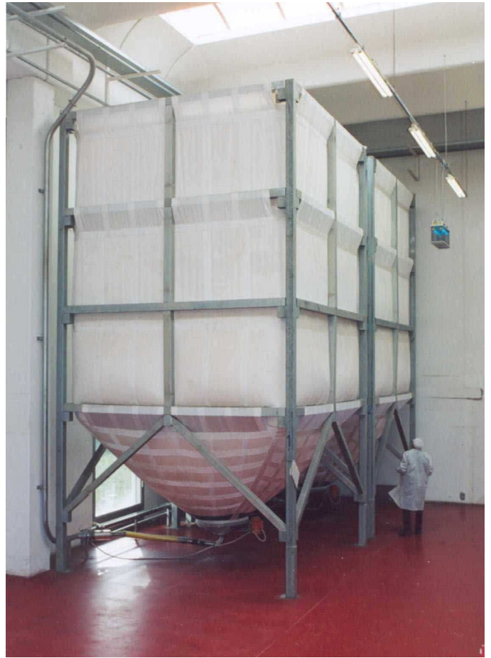
Fabric silos in Trevira type high tenacity fabric suitable for internal storing of powder products
